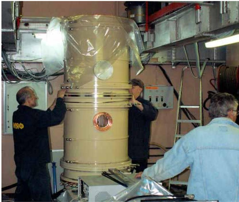
Fig.(7.5)1. Section of the accelerating structure in an upright position.
