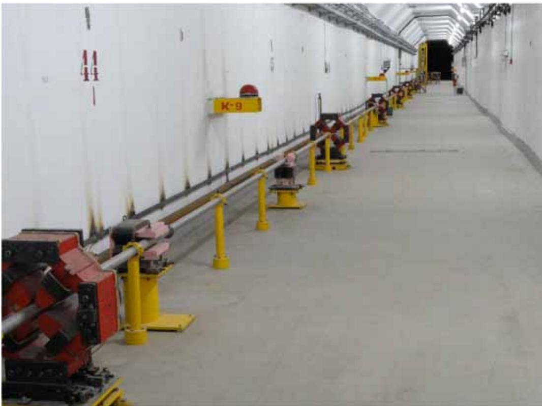
Fig. (5.3)5. General view of channel to VEPP – 2000 with magnetic elements, cable trays and ground loop.
