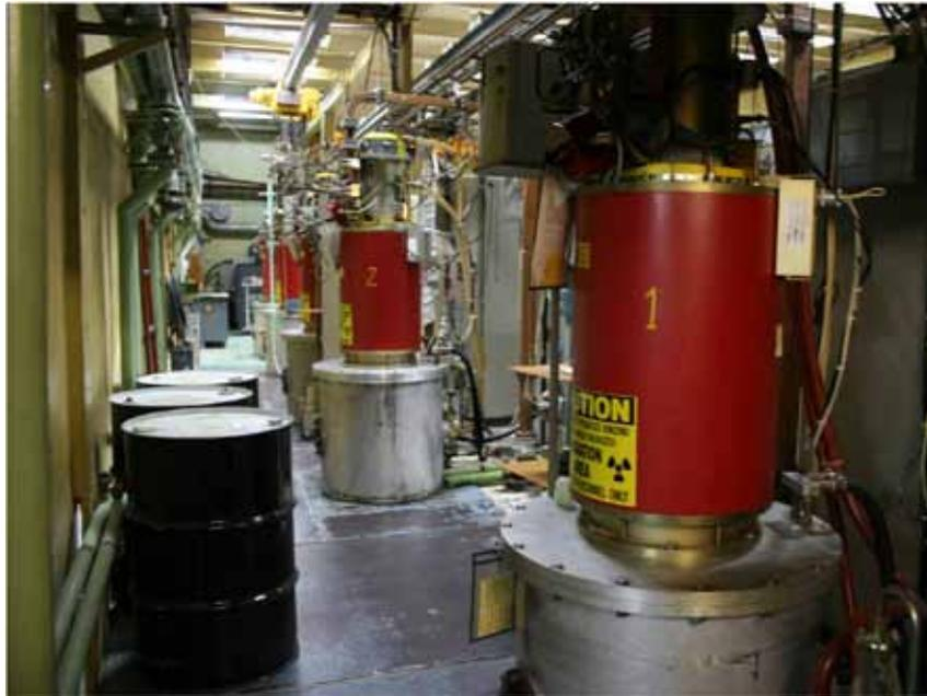
Fig. (5.3).2. Klystron preinjector gallery of IC VEPP – 5 with all klystrons.
