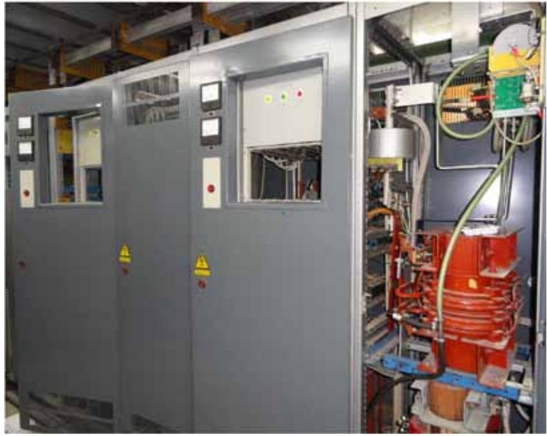
Fig. (5.3)10. Reversible current power supplies IST for IC channels.
