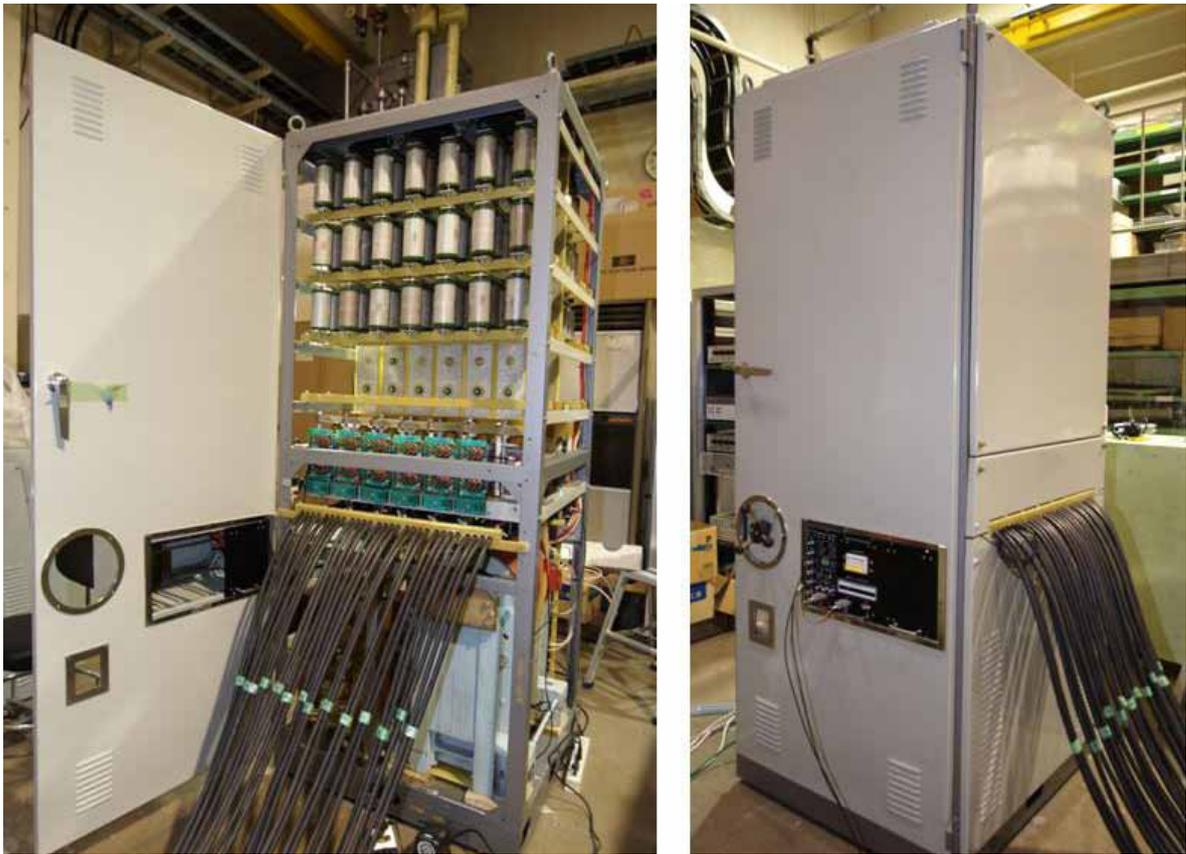
Fig.(5.13)1. Power supply of the conversion magnet.
