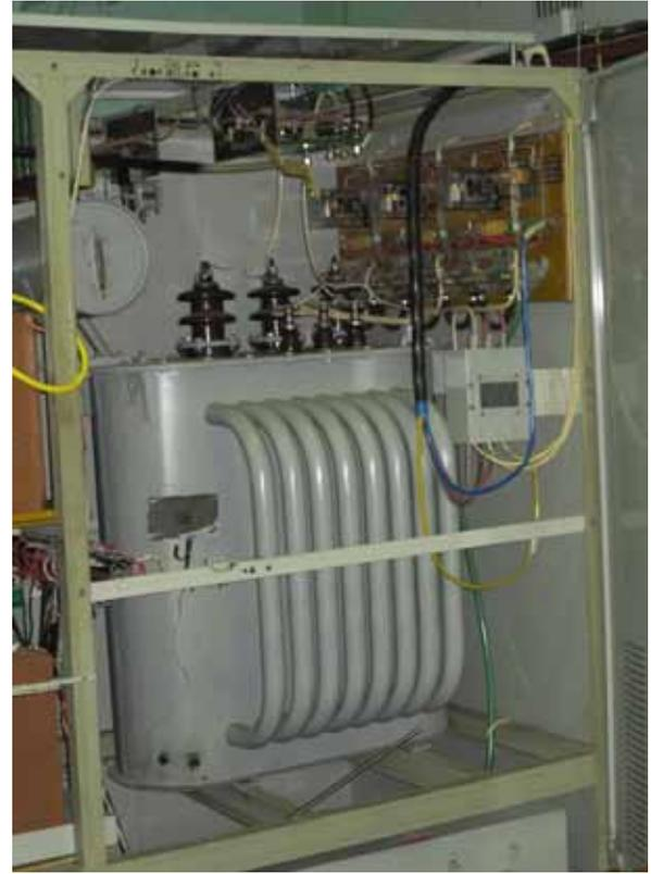
Fig.(5.11)4. High voltage regulable rectifier with a capacity of 100 kVA.
