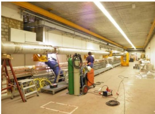
Fig. 5.10.5. Mounting of cryogenic equipment in hall of injector 1.
