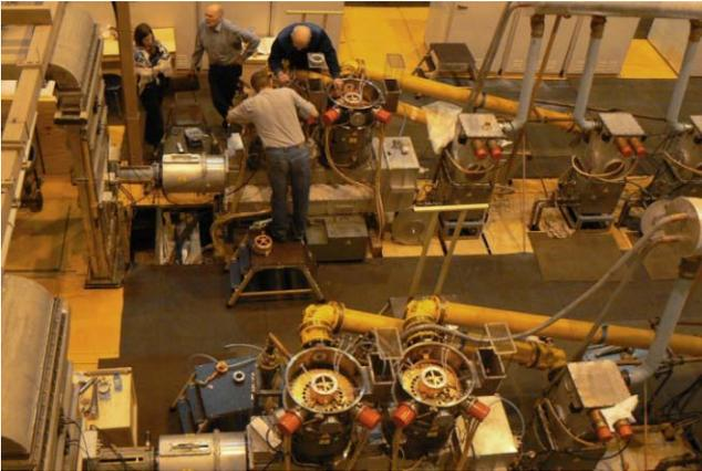
Fig. 7.9.1 Panorama of generator hall of complex Sibir-2 during replacement of tubes.
