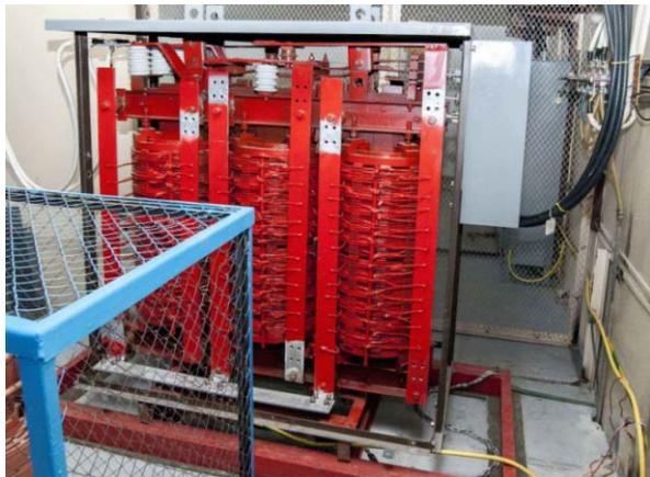
Fig. 7.6.2. Transformer and diode bridge (right) of anode voltage boost.
