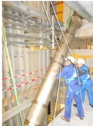
Fig. 5.10.6. Mounting of pipeline in shaft of XFEL building.
