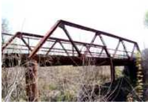
Figure 3.11: Warren Truss [63]
