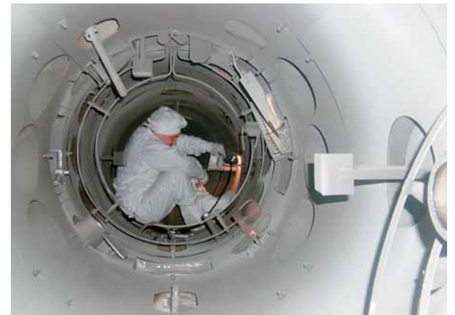
Inside the GDT vacuum chamber
